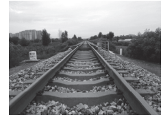
铁轨下面铺放枕木
